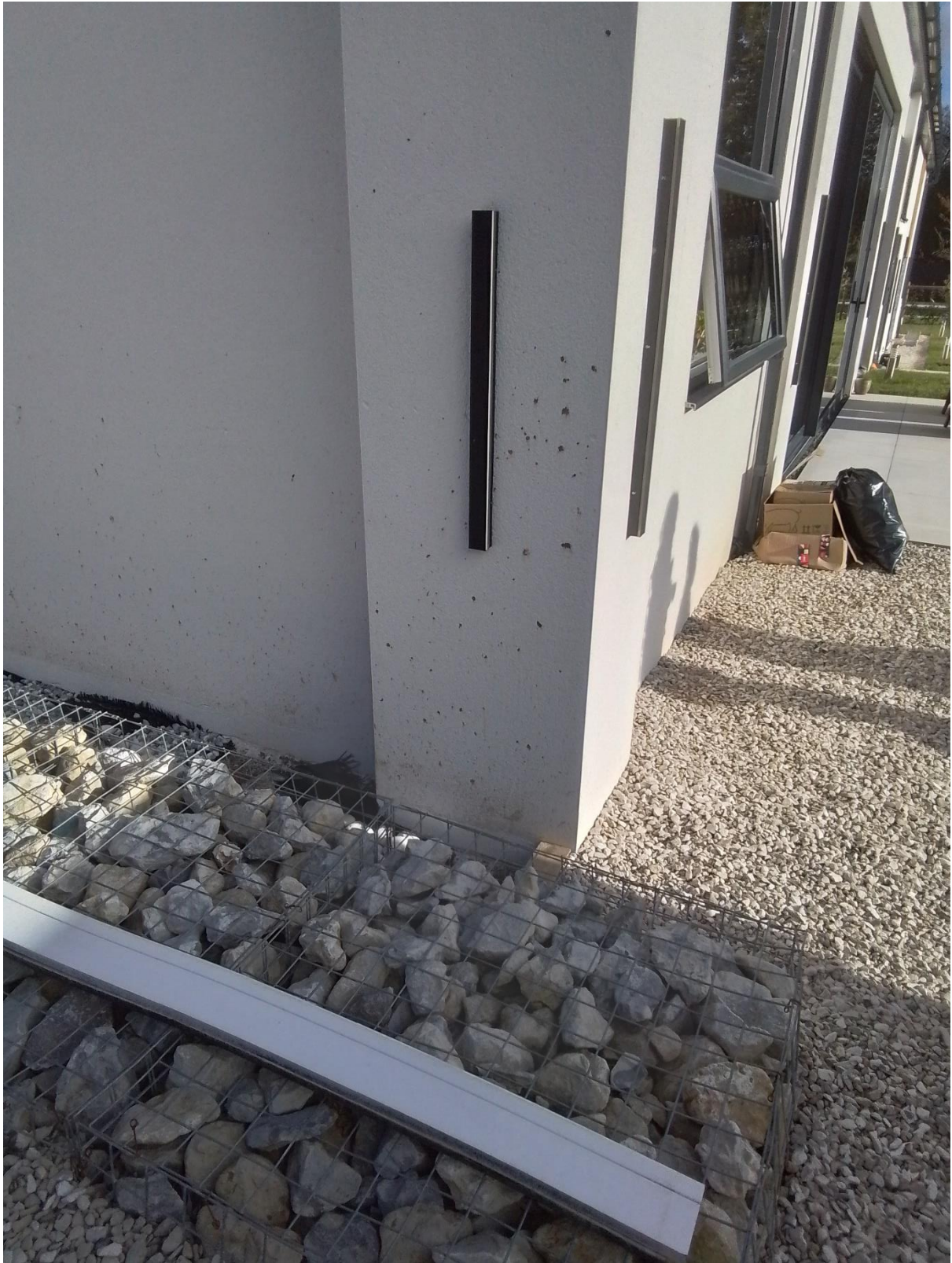
View looking along the front South Elevation
