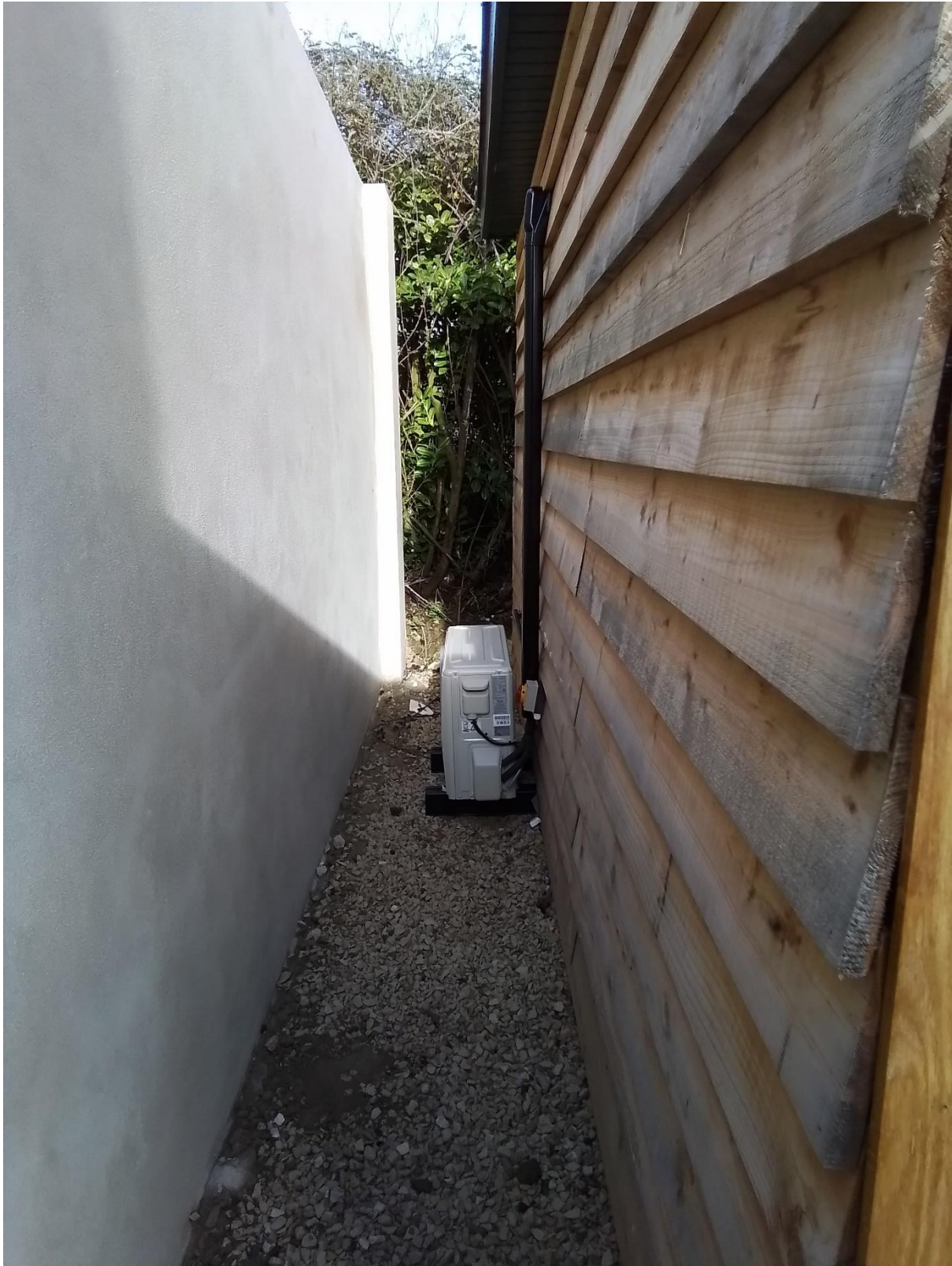
Space between outbuildings with air con West
