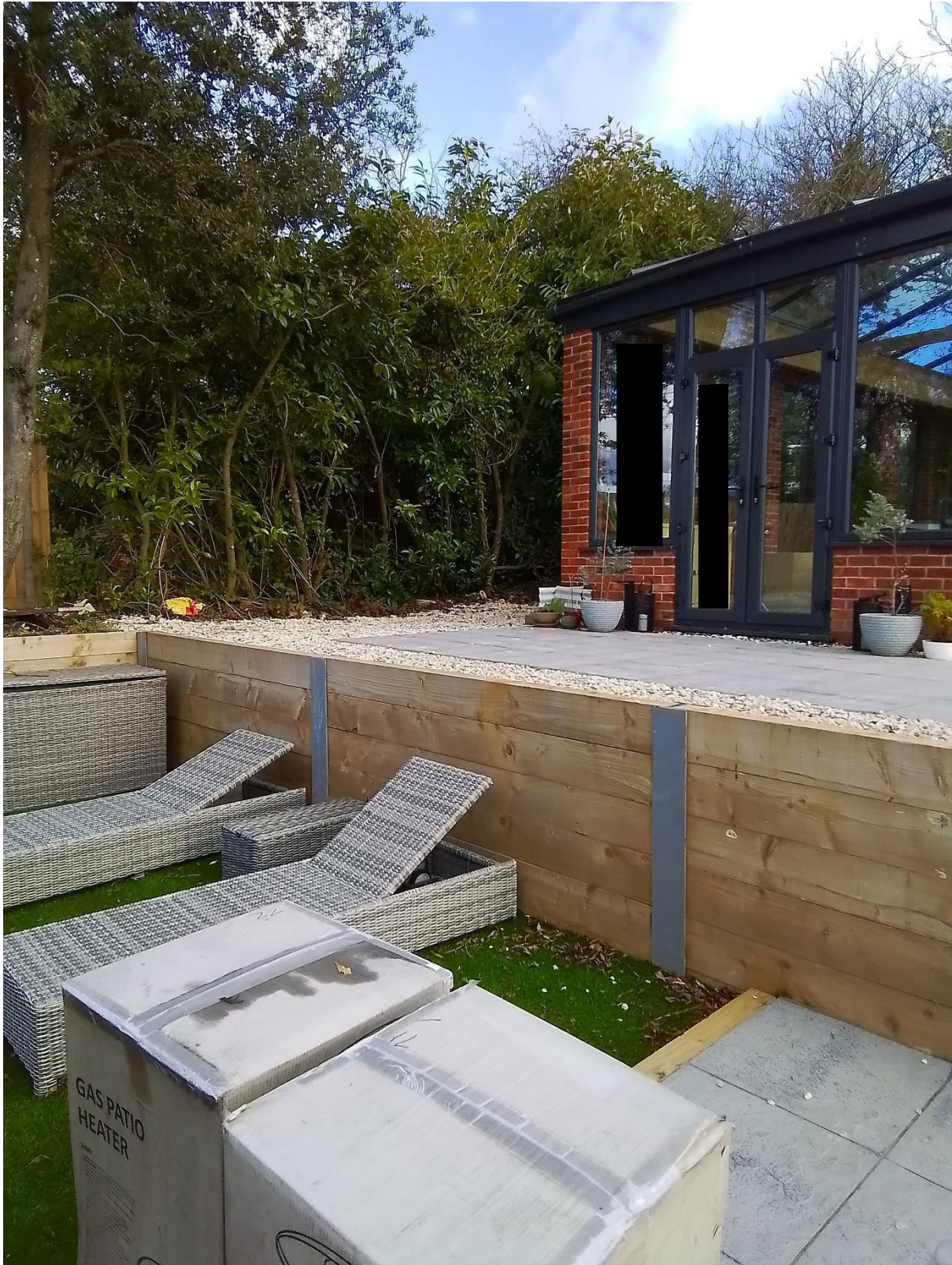
Retaining wall and view of greenhouse
