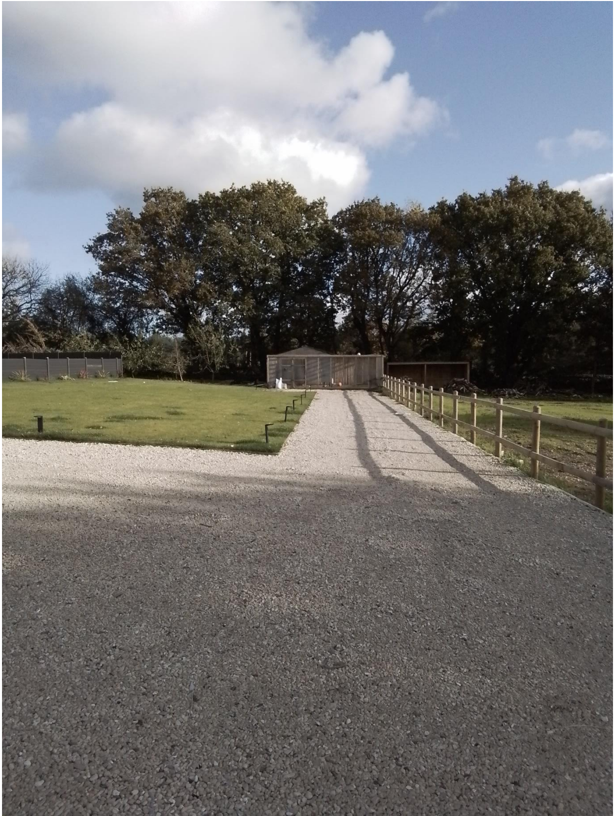
View of second driveway W to E looking E
