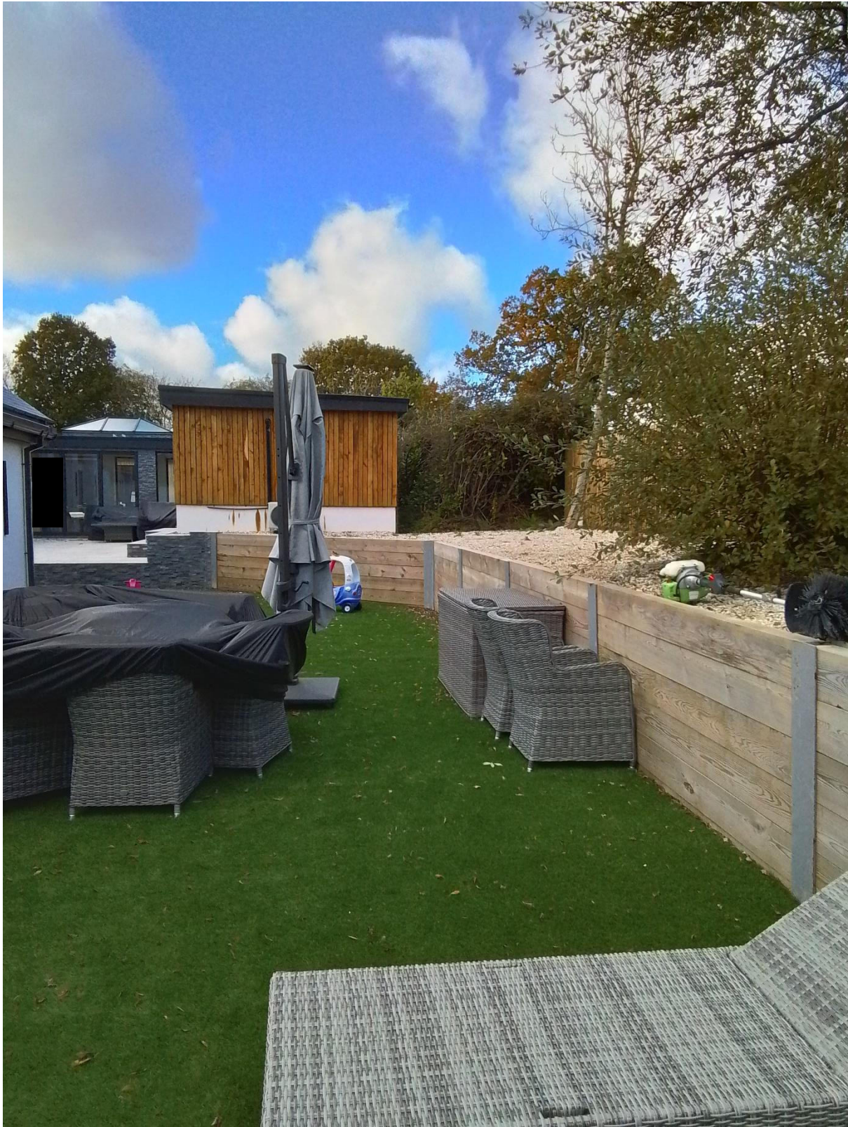
Retaining walls on Northern side
