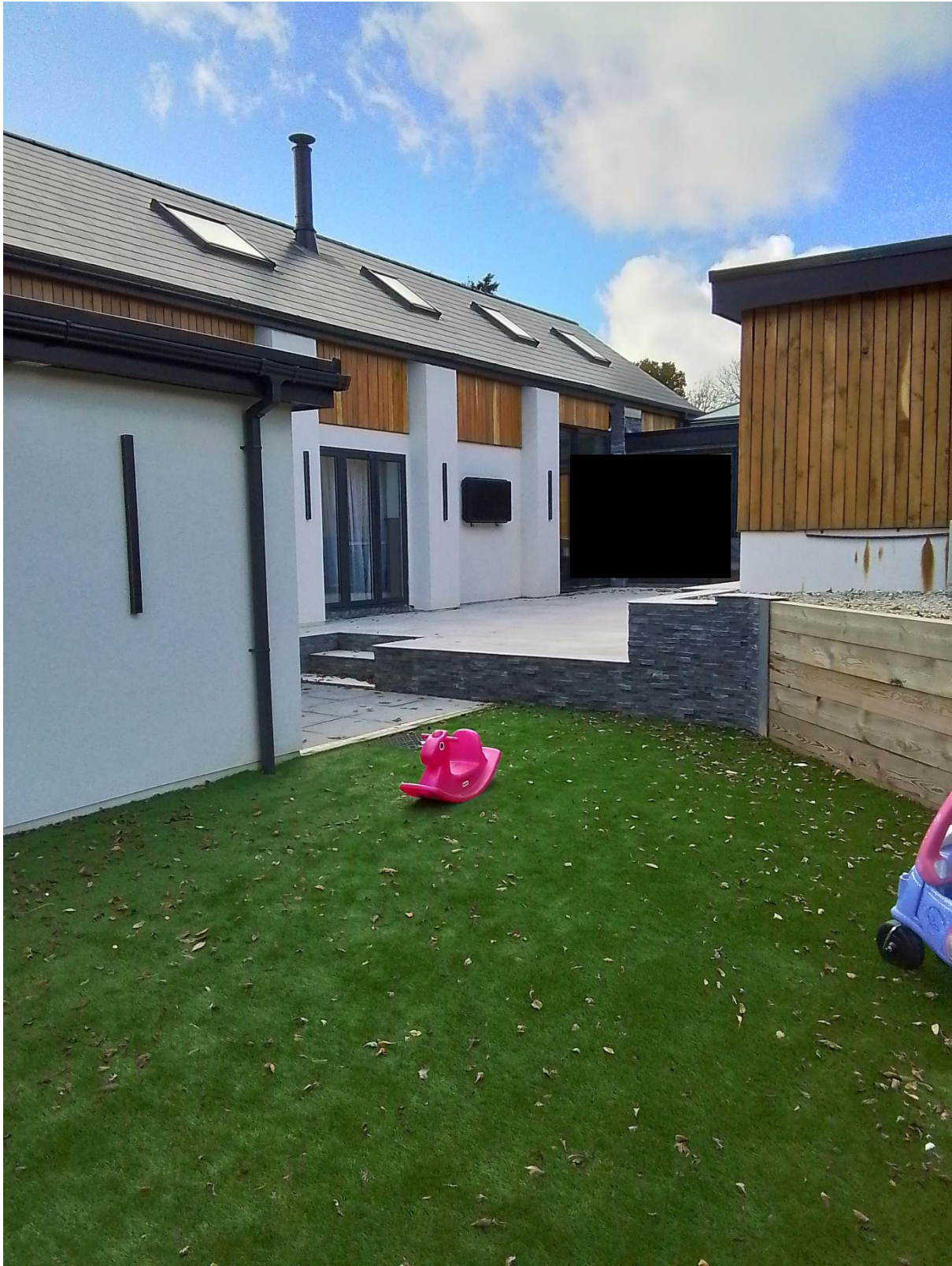
Roof lights on North Elevation
