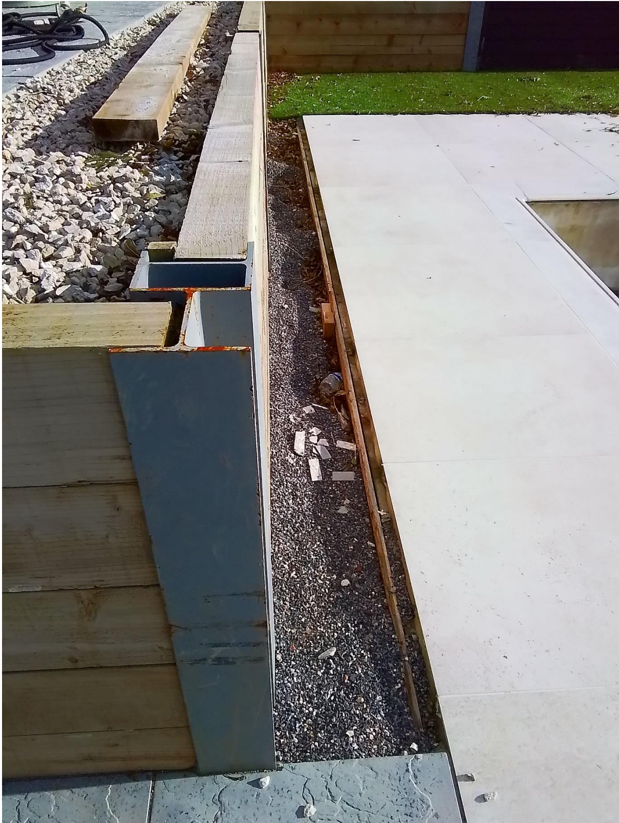
Retaining wall adjacent to swimming pool
