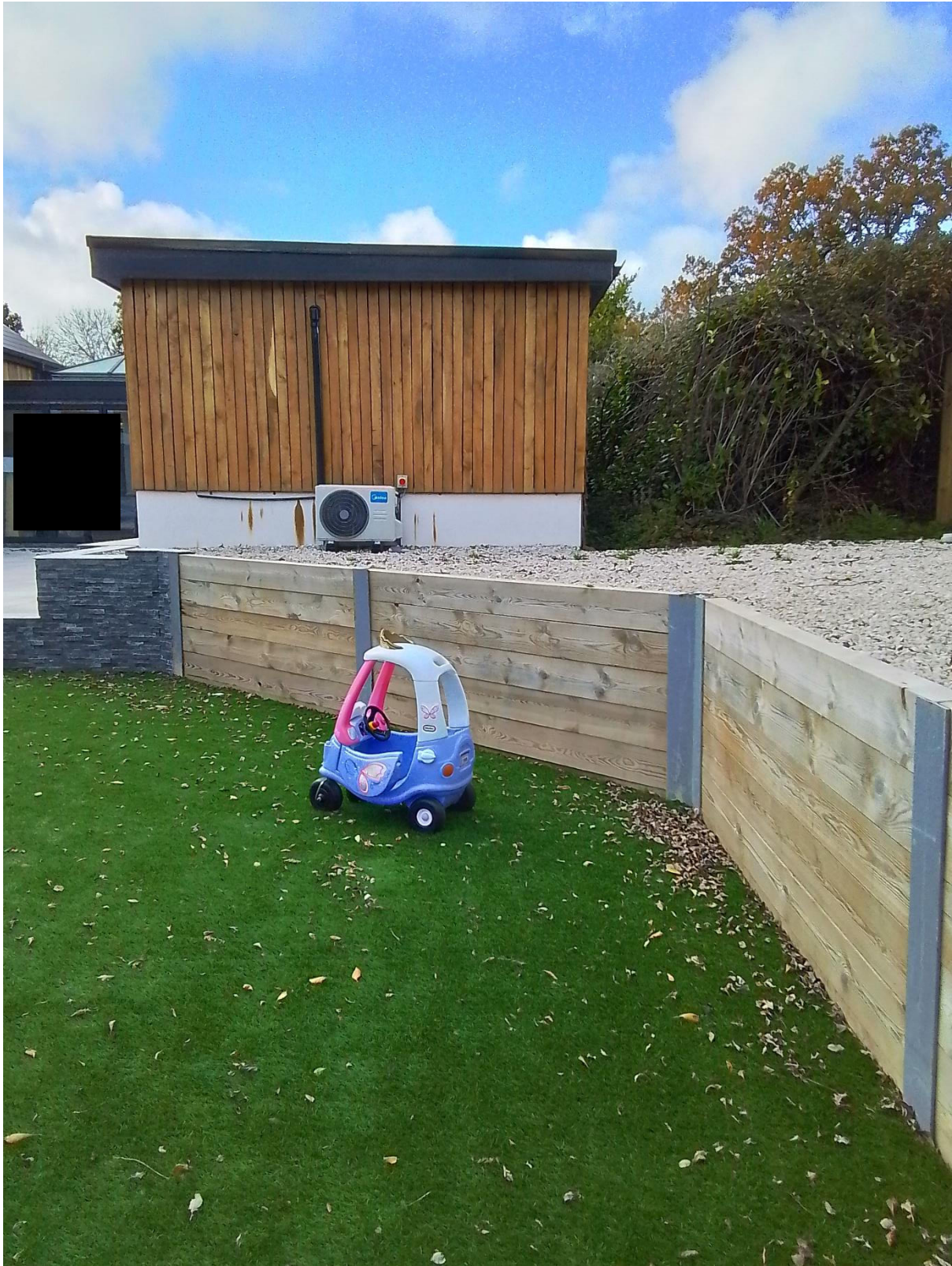
Retaining wall and end of outbuilding extension NW
