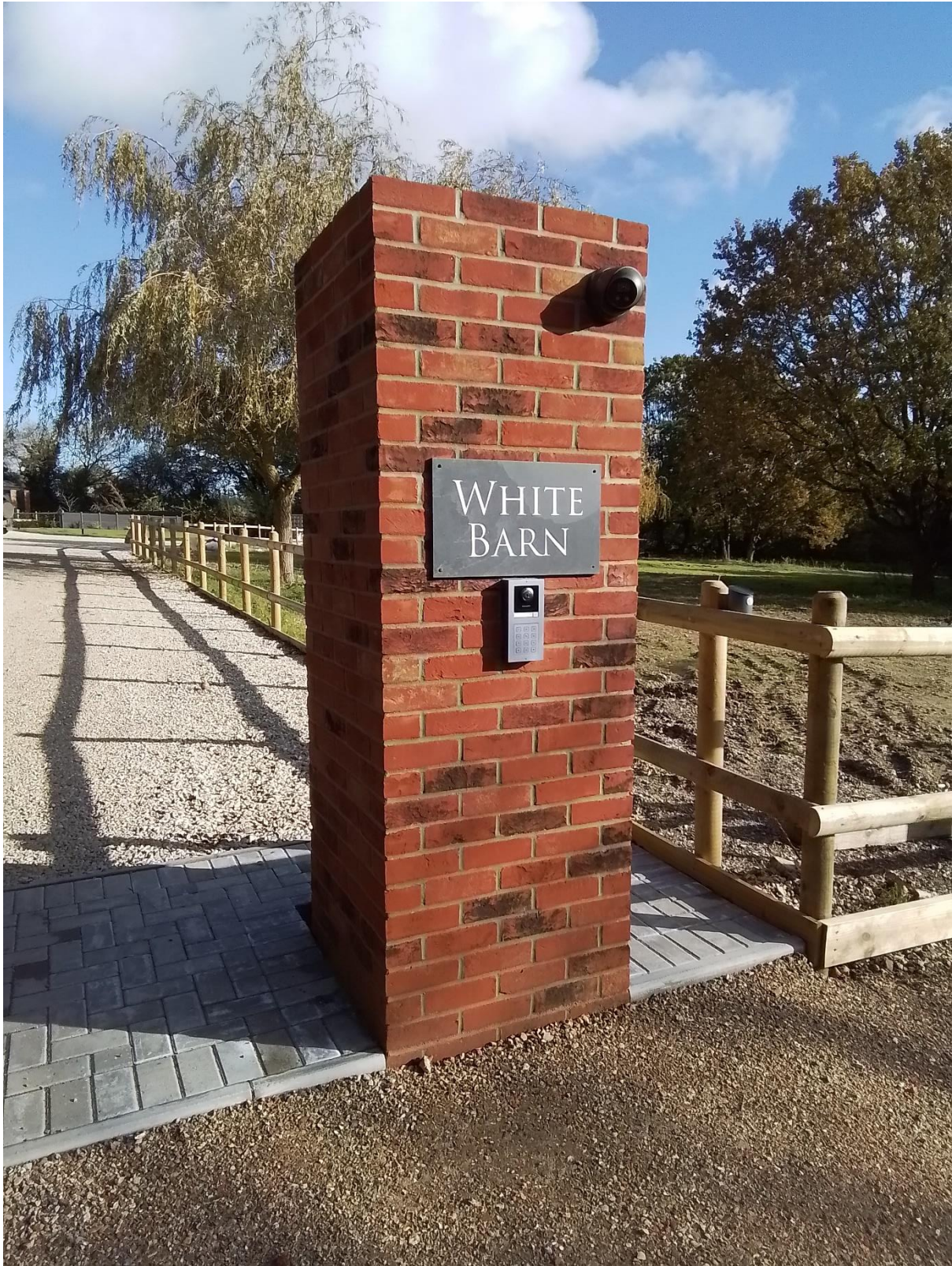
Pillar at entry point and drive looking NE
