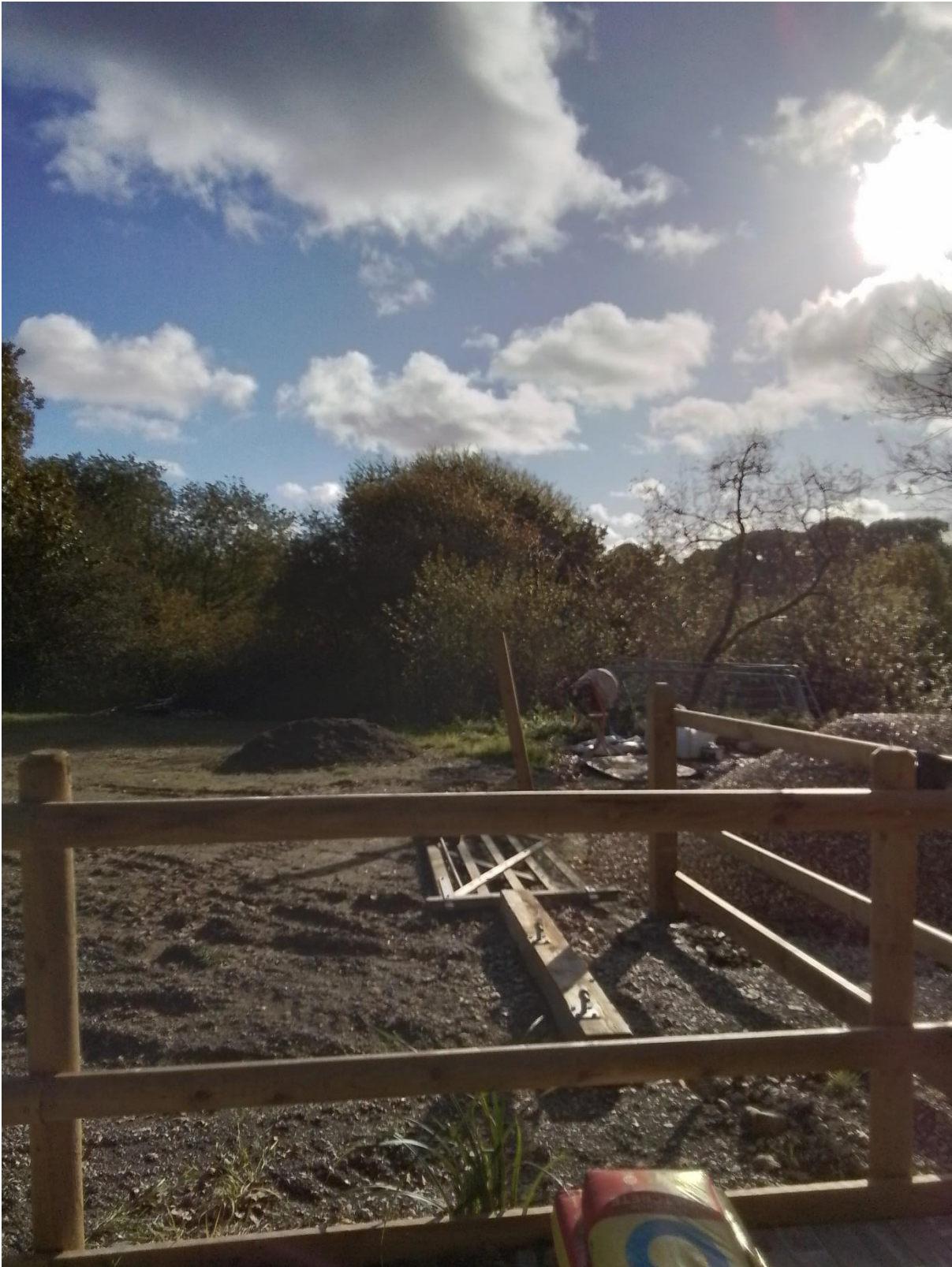
View looking SE from driveway
